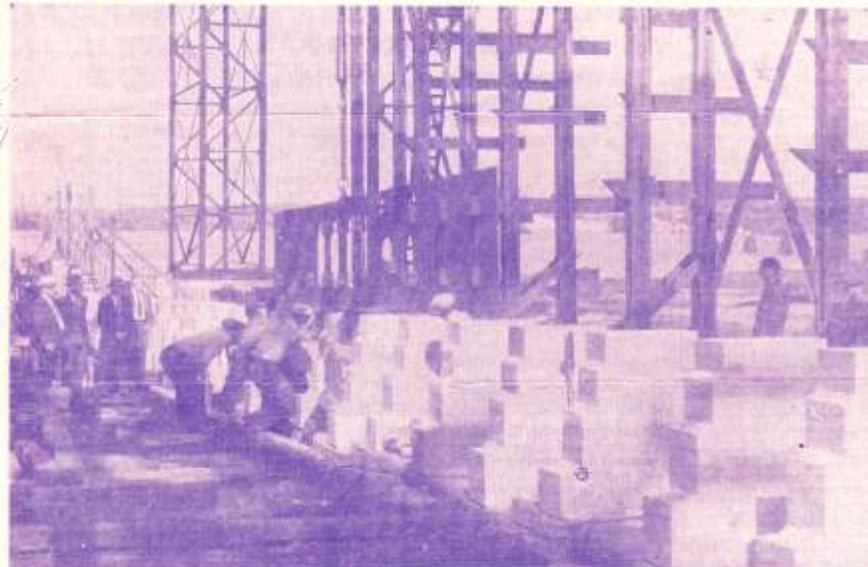
Workmen are pictured placing in position the first vertical keel plate for the United States submarine Skipjack at the shipyard of the Electric Boat Co. at Groton. The keel-laying ceremony took place yesterday in the presence of navy officers and officials of the constructing company, and several are seen standing by.
